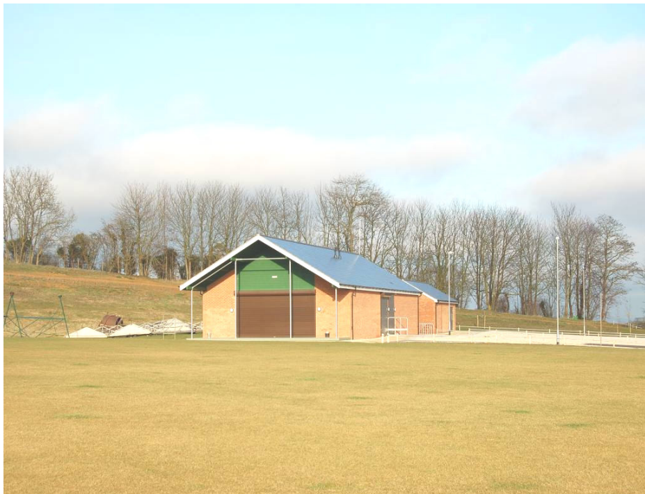
Figure 16 Cricket pavilion and store looking south-west
