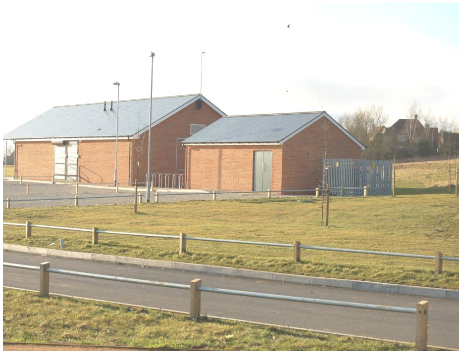
Figure 10 Cricket pavilion and store looking west from south side of site access road.
