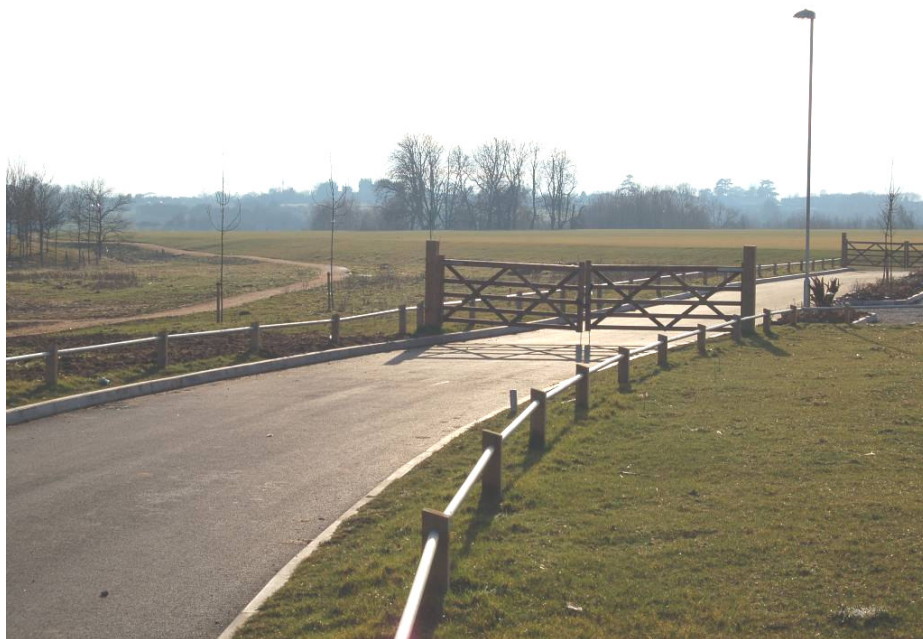
Figure 8 Access gate to main car park from Stanford Road entrance
