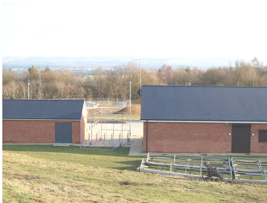
Figure 20 Space between store (left) and pavilion (right) looking south
