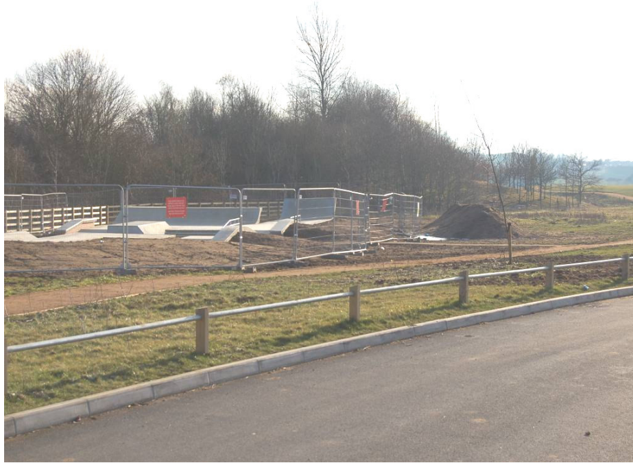
Figure 7 Skate park looking south, from site access road
