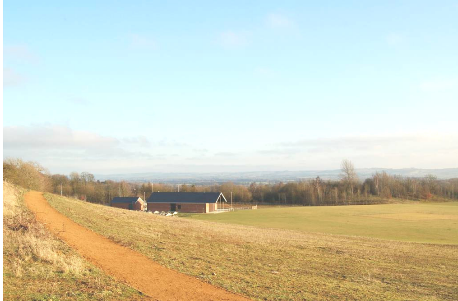
Figure 1 Path leading south-east towards cricket pavilion and store
