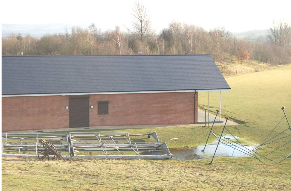
Figure 21 View looking south towards north elevation of pavilion and south perimeter boundary
