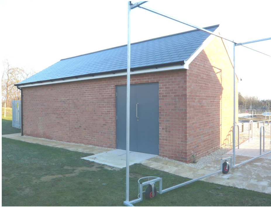
Figure 25 South-east corner of store
