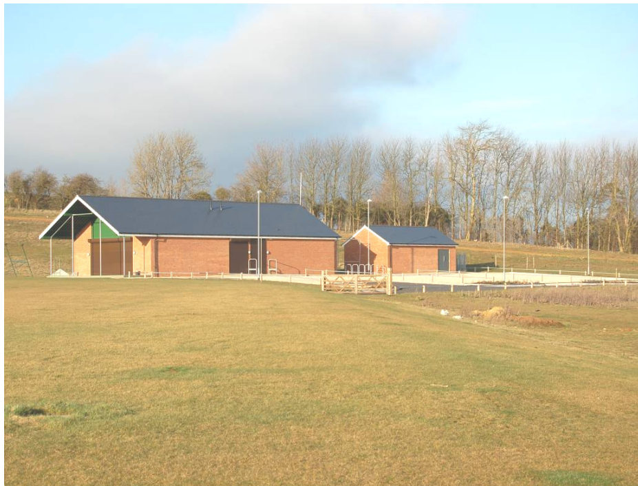
Figure 12 Cricket pavilion and store looking north-east from cricket pitch
