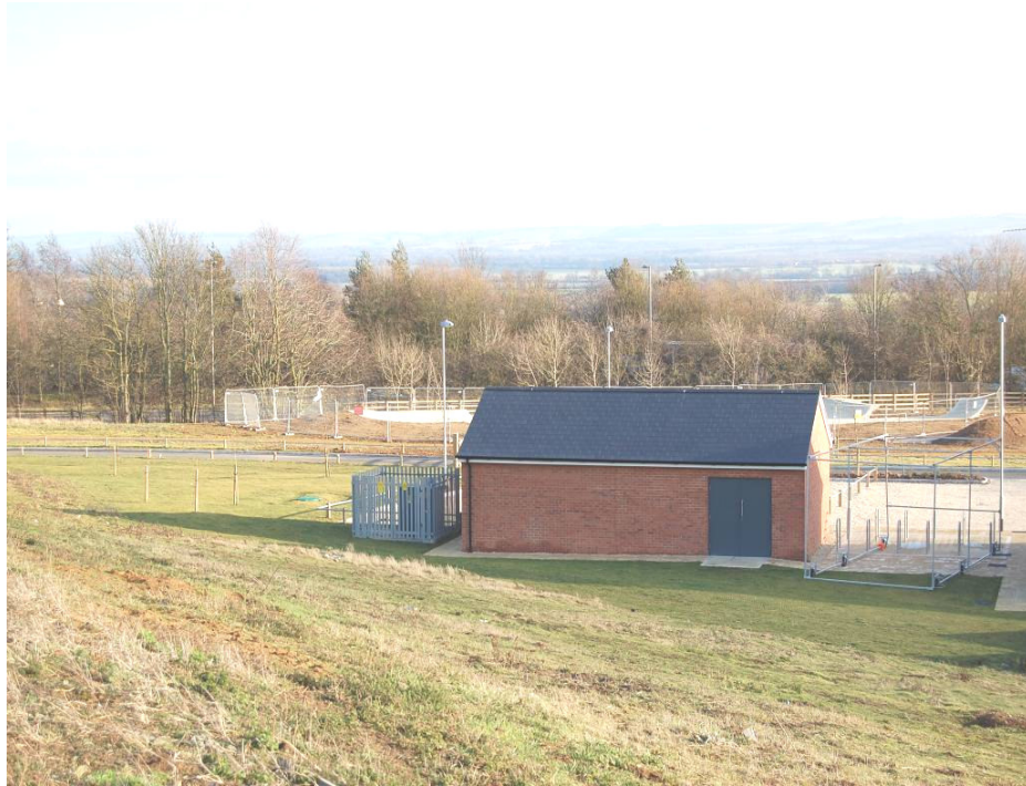
Figure 19 North elevation of store building
